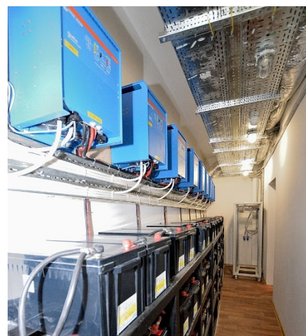
8. - 90KW (180KW peak) of off-grid power units providing a hard-bypassed central single phase backup inverter solution for an entire film post-production facility. - No I.T. UPS could cope with this. - System comprised of Nine Victron Energy Quattro
